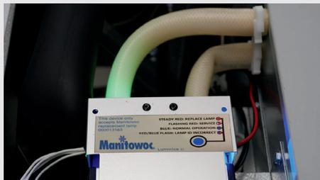
*The LuminIce II space-saving design fits inside the ice machine so existing exterior clearances are not impacted. In addition, power for the unit is supplied through the ice machine's internal electrical supply so outlet space is conserved.*
